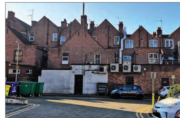
Rear of 39-51 Green Lane
