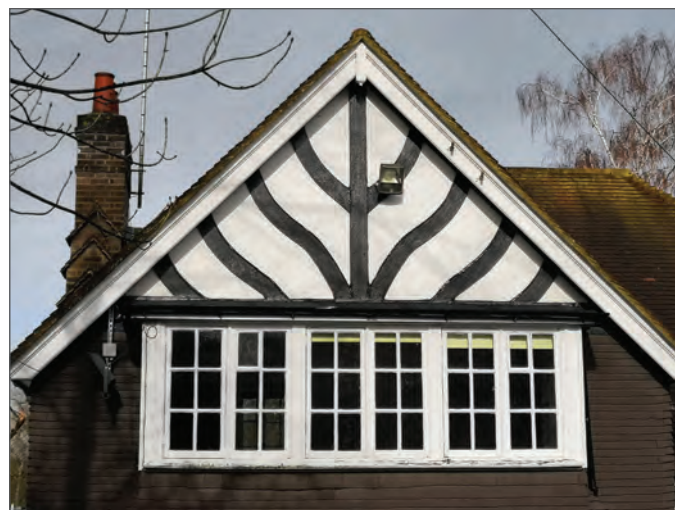
Half-timbered gable, hipped roof, brick chimney stack
