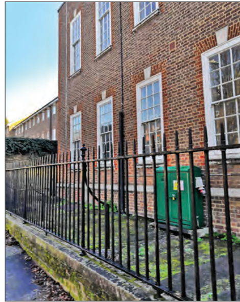
Wrought iron railings
