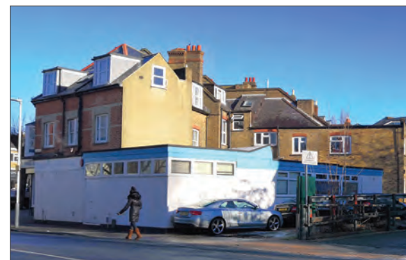
Rear of 3-27 Maxwell Road shops
