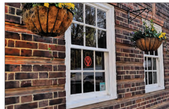
Six over six timber sash windows
