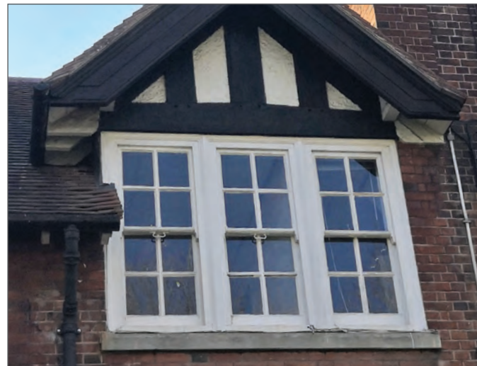
Six over six timber sash window with horns
