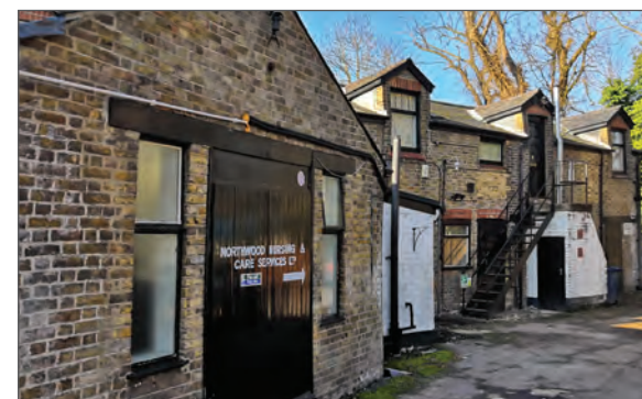
Outbuilding, rear of Green Lane
