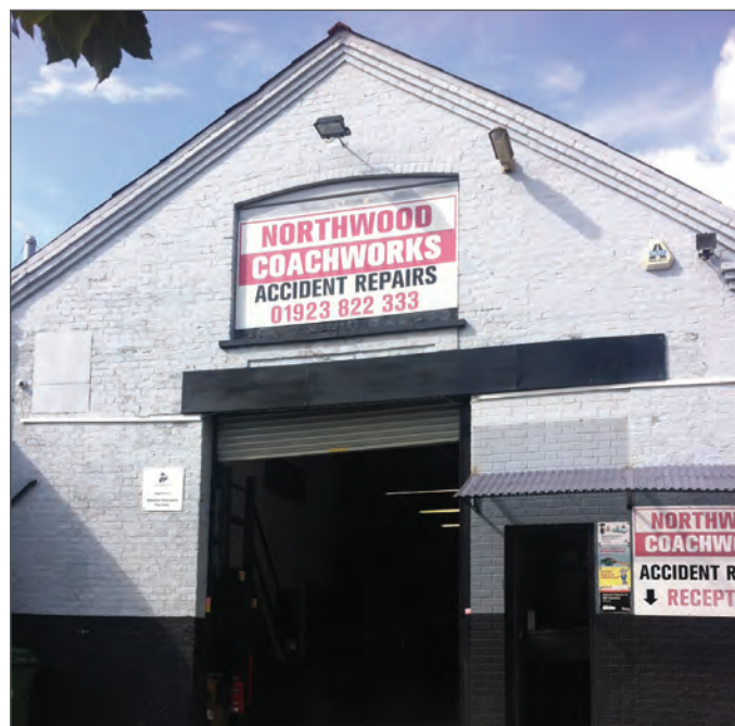
Railway sheds behind Station Approach
