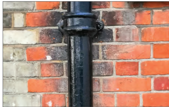
Cast iron downpipe
