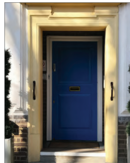
Original recessed door and stone door surround
