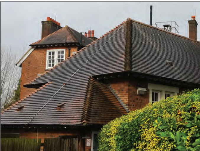
Hipped roof with cat slide
