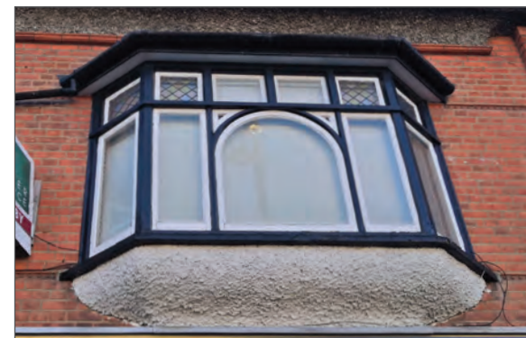
Ogee and dormer windows
