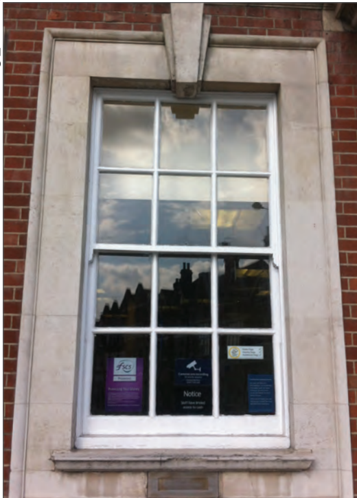
Six over six timber sash with horns stone architrave
