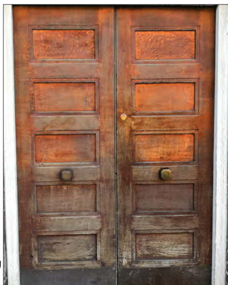
Art Deco five panel door with original door furniture
