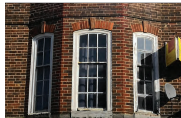
Bay window with small paned sashes
