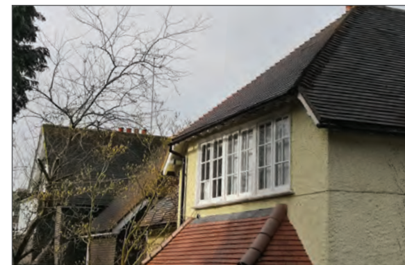
Three quarter hipped roof
