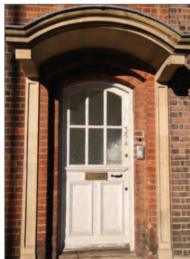
Curved stone door hood and original timber door
