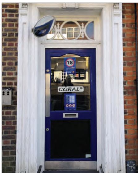
Neo-Georgian painted timber door surround
