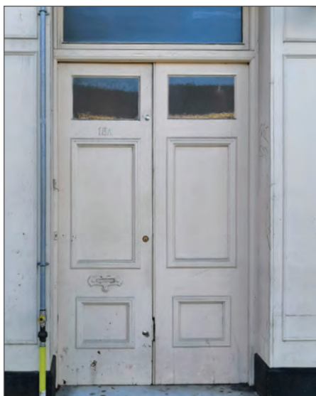
Timber double door, door light
