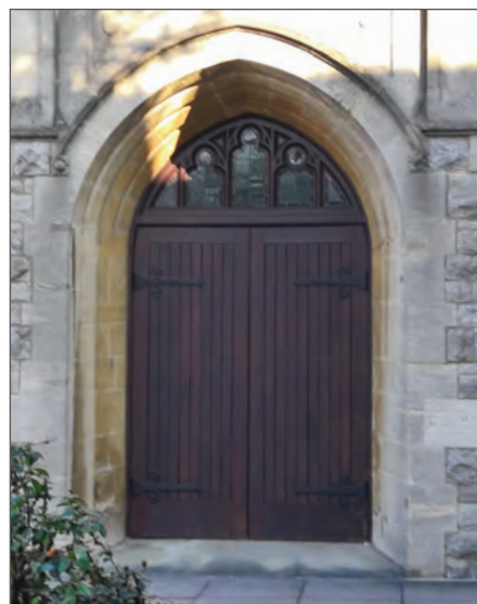
Pointed arch opening for wooden door and door light
