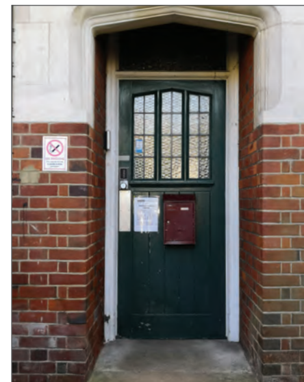
Recessed half glazed timber door under Tudor stone porch
