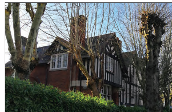
Police Station, 2 Murray Road, north elevation
