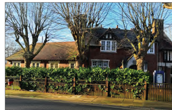
Police Station, 2 Murray Road, east elevation
