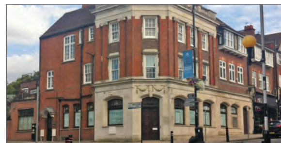
Former NatWest Bank, Green Lane
