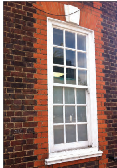
Nine over nine timber sash with horns
